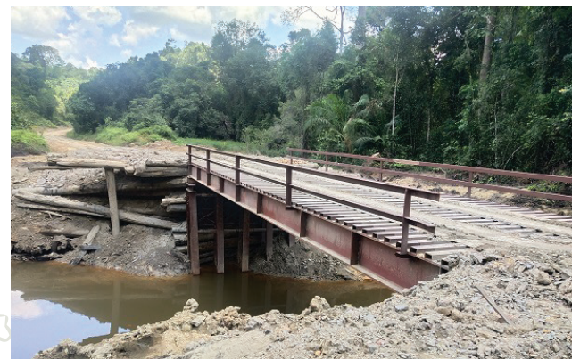
Sg. Linei Putih I-beam bridge
