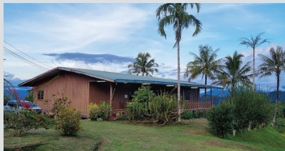
Staff quarters at camp.
