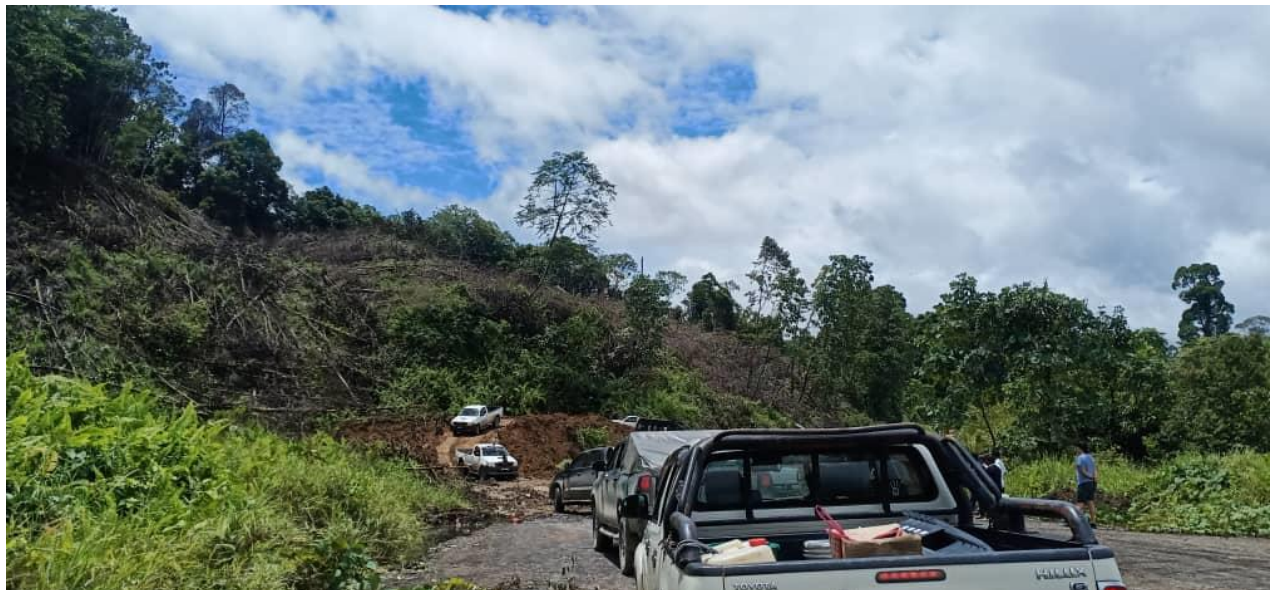
Work-in-progress. Passable by 4- wheel drives by mid-day on Monday, 14 September
