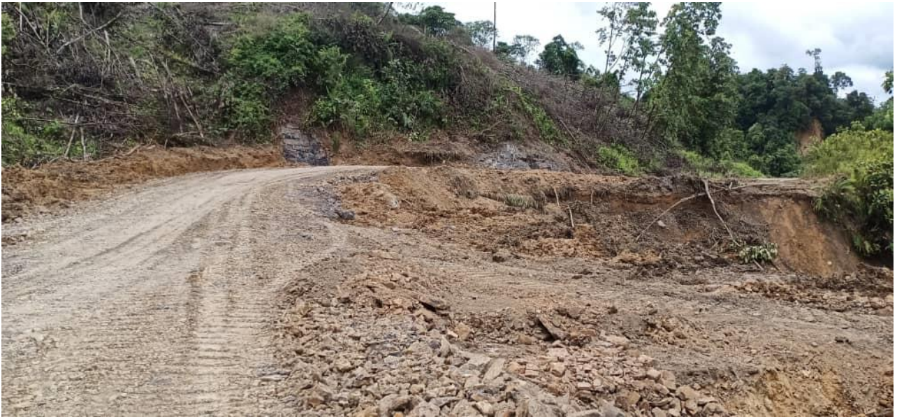
Stretch of road fully restored by mid-day on Tuesday, 15 September
